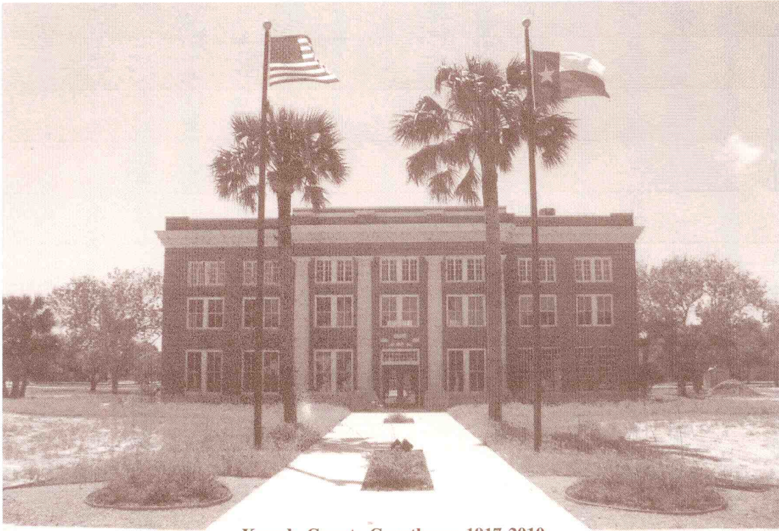
Kenedy County Courthouse 1917-2010
